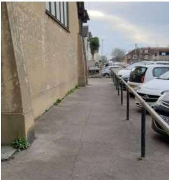
Figure 3 - From the north-western corner of the church, looking southwards.
